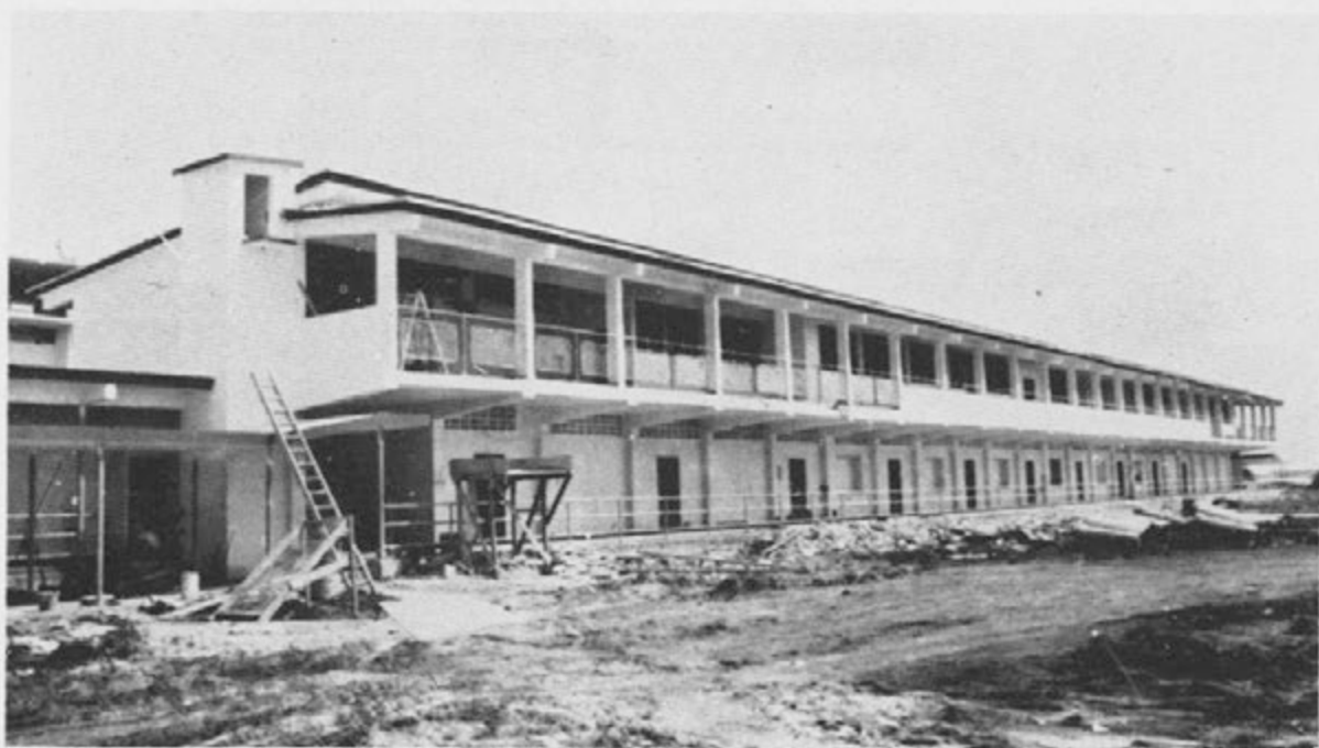
Central American and Caribbean Village under construction.
